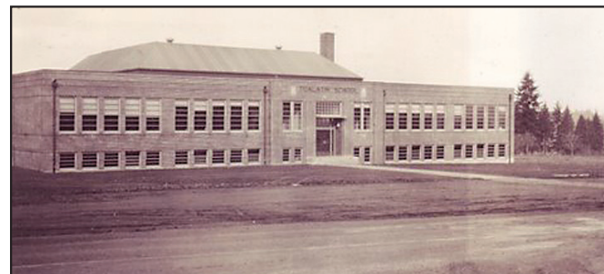
Tualatin Elementary School was state of the art in its time. The school board borrowed the plans from Collins View School, and the bricks were hauled in from Willamina. Teachers would open the windows on warm days with a long pole with a hook on the end.
