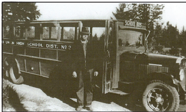
August Ite, Ite and Ite School Bus Services stands in front of Reo Speedwagon School Bus he sold to Tualatin Fire Department who converted it into fire truck #2 below
