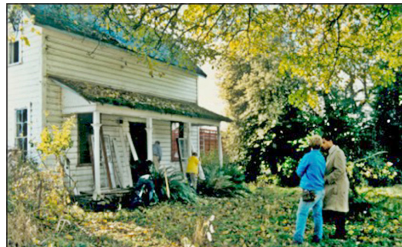
Dismantling the Hedges house and numbering every board
