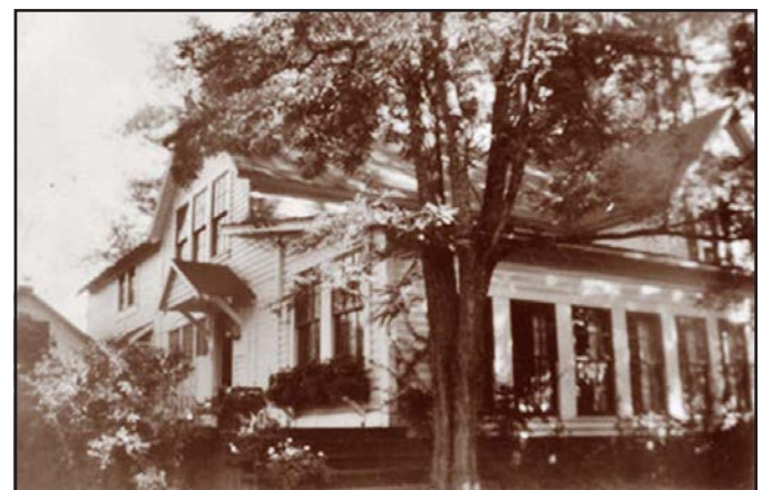
The Sam Galbreath house was close to the Tualatin river on the south side. Sam was the son of Oregon Trail pioneers Samuel and Sarah Galbreath. Sam was married to Janie McE Graham of Grahams Ferry fame.
