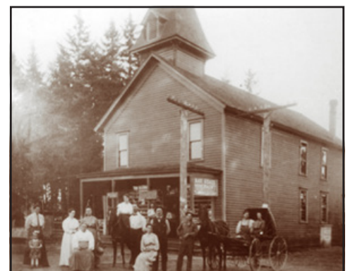
The Smith family had a sawmill in the current city park. They built this store on the corner of Boones Ferry and Tualatin Road. The store was operated by Lizzie Smith Robinson and her husband Newt. The store was moved east in 1912 and the current brick store was built on the spot, using bricks from the Smith brickyard which was down past Clark Lumber Co.
