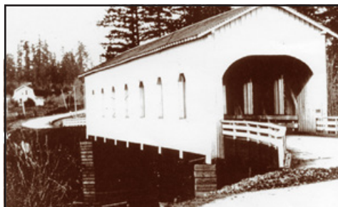
Taylor's Ferry bridge on highway 99. Bridges were covered to keep the bridge from rotting out, and also it's said that horses would not want to cross if they could see the river.
