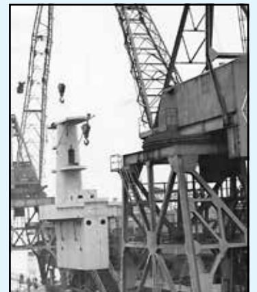
Moving superstructure onto ship with cranes.
