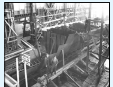
Ships were built from hull up with sheets of iron plates either riveted or welding together.
